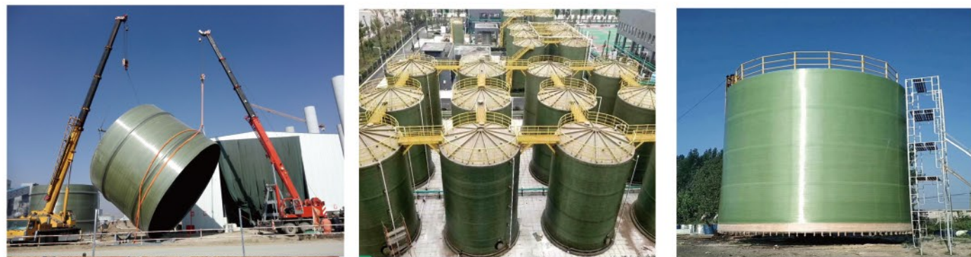
现场缠绕大型罐 SITE WINDING MAX TANK
