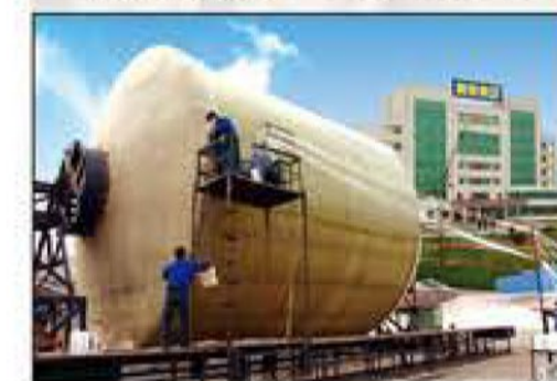
现场缠绕大型罐 Site winding max tank
