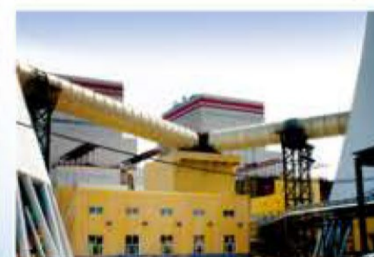
哈爾濱第一熱電廠烟塔合一工程 Fume pipe and tower syncretic project in Habin 1st Thermal power Plant
