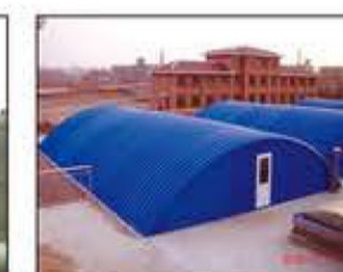
污水池盖板 Cover plate of sewage pool
