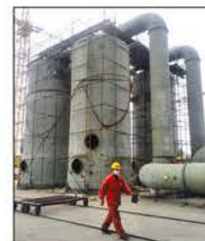
生物罐 Biological tank
